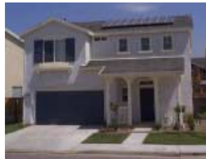
Figure 1 Roof Mounted PV System
